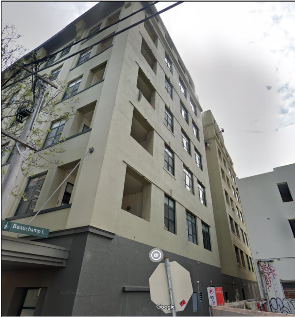
Figure 2: Photo of the Eastern Elevation of SP 57988 from the corner of Reservoir St and Beauchamp Lane showing central lightwell and windows and balconies to the eastern façade (existing development on the DA site on the right) (Source: Google maps)
